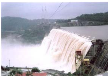
Dam over the Narmada river (India)
