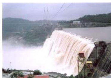
Dam over the Narmada river (India)
