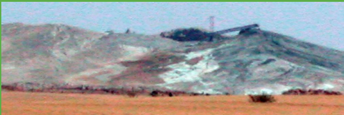
Radioactive tailings (from COMINAK uranium mills) stored out in the open Photo by CRIIRAD, December 2003
