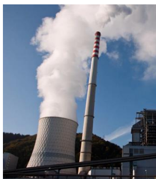
Lignite power plant in Sostanj – TES
